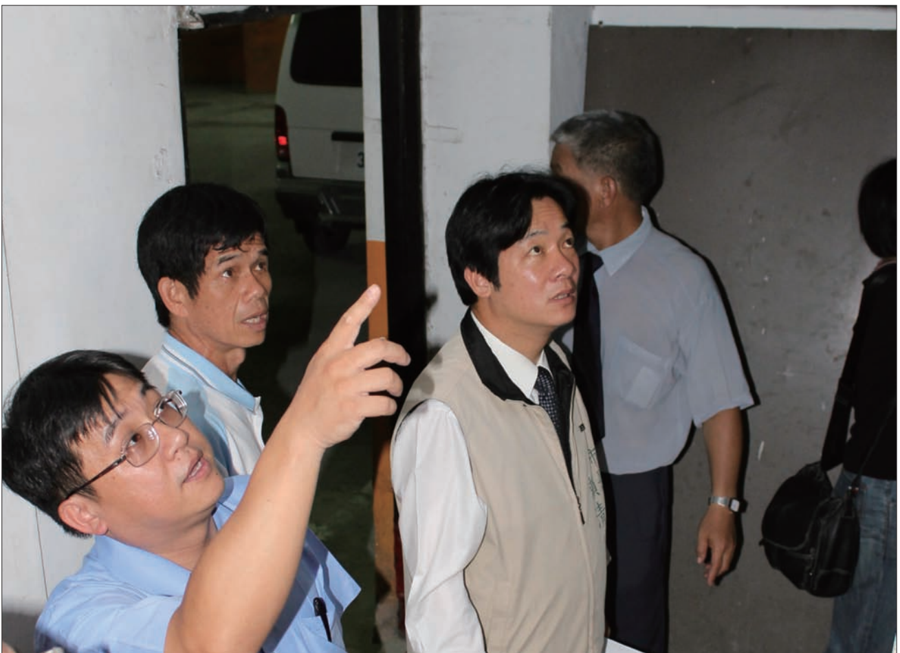
© On-site survey of building damage
