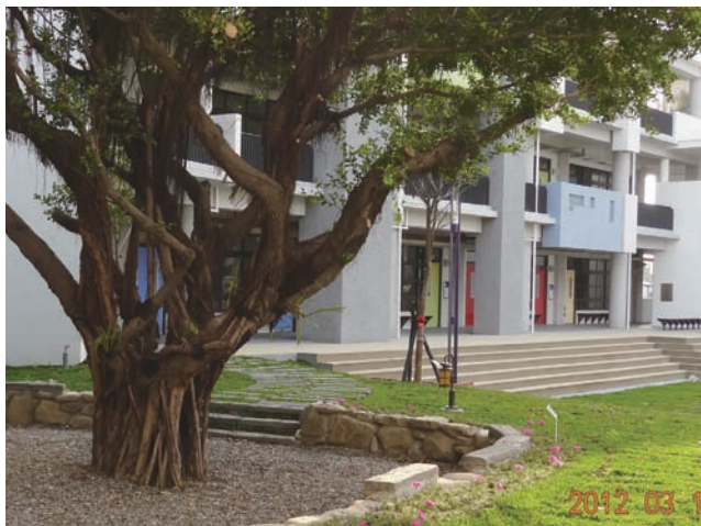
◎ North District Daguang Elementary School
