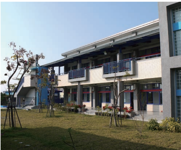
◎ Du Jia Elementary School Building Reconstruction Works
