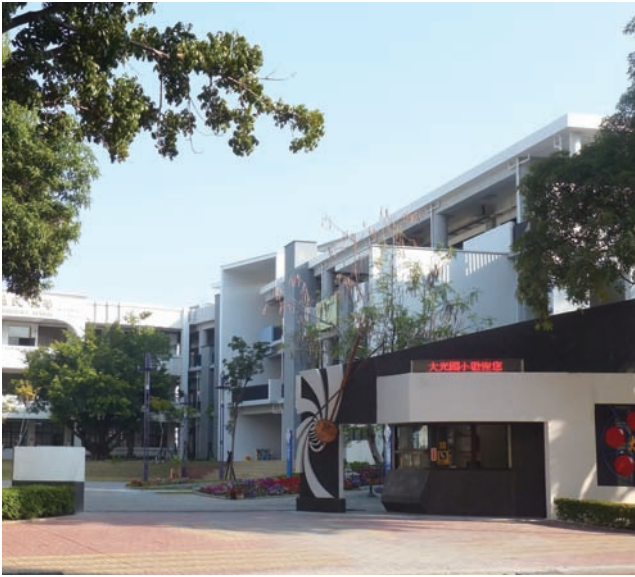
◎ Tainan Daguang Elementary School classroom demolition and reconstruction project
