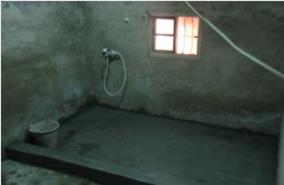
The walls in the bathroom was under construction
