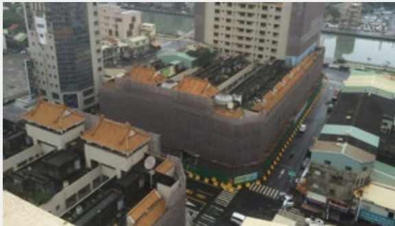
The former China-Town Mall (the west side of Jinhua Road)
