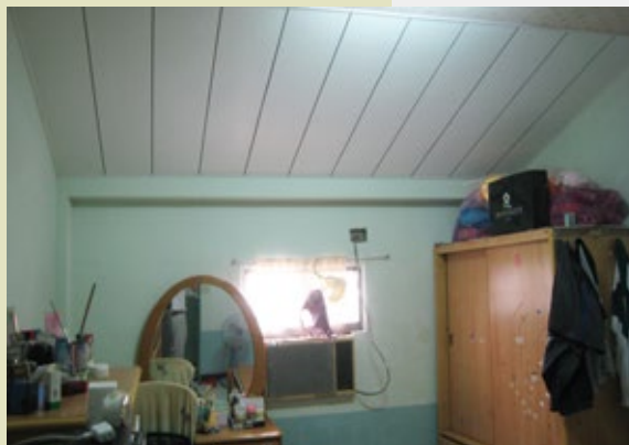
The new ceiling and walls (After repair and repainted)
