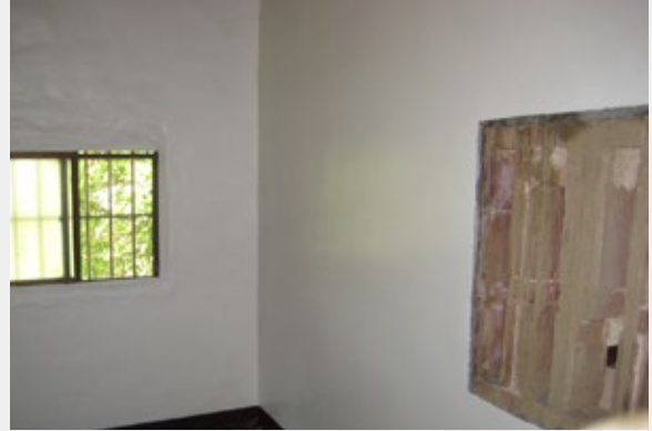
The walls were plastered and repainted
