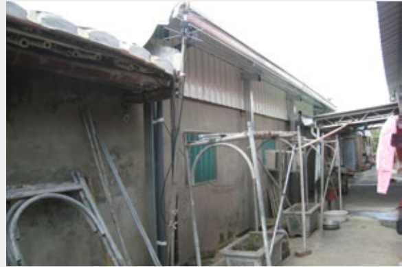
Light Gauge Steel Roof (after construction)
