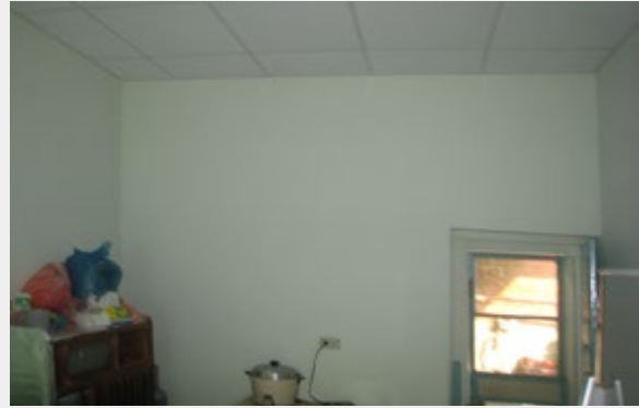
The new ceiling and the repainted walls (after repair)
