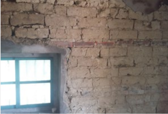
Inside the rammed earth house (before repair)
