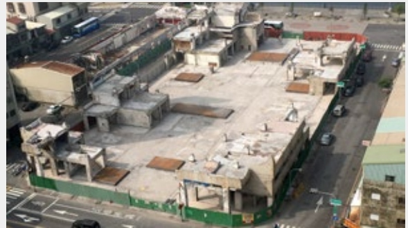
Completion of the demolition work (the west side of Jinhua Road)
