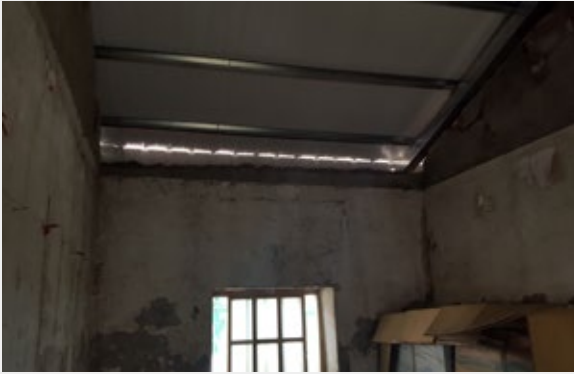
Installing the new ceiling (under construction)
