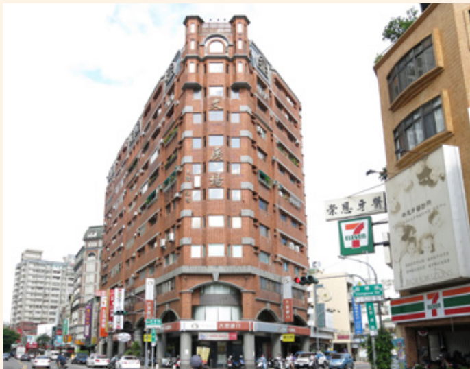
► Wenhua Guangchang Building in East District (before renewal)
