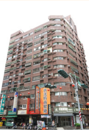
▶ Jiaxi Wanchao Building in Yongkang District (before renewal)
