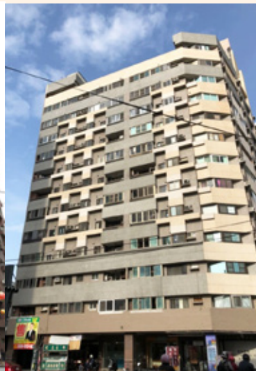
▶ Jiaxi Wanchao Building in Yongkang District (after renewal)
