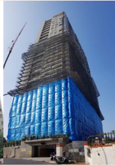
▶ Guojia Sinjing Building in East District (under construction)
