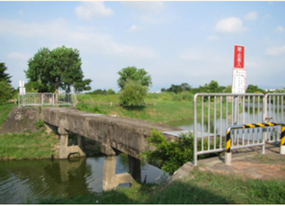
▶ The bridge at the Yuejin Harbor Park will be renovated
