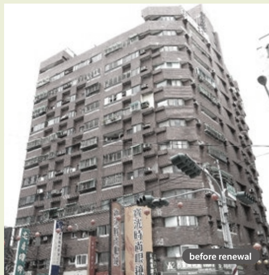
Jiayi Wanchao Building, Yongkang District
