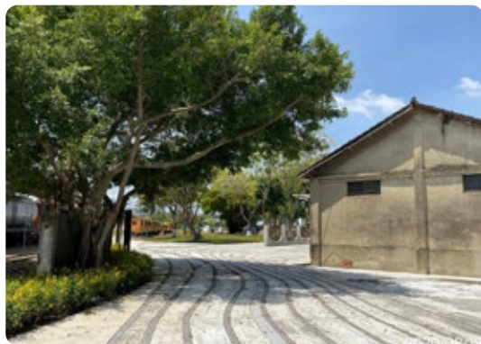
Results of second stage work on the Sinying Railway Scenic Park
