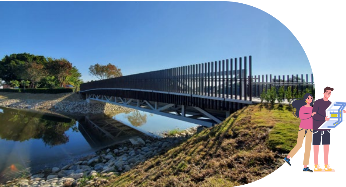
People are encouraged to visit the box bridge over the river at Yanshuei's Yuejin Harbor and see the magic of the water in person
