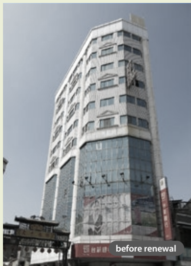
Ximen Finance Building, West Central District
