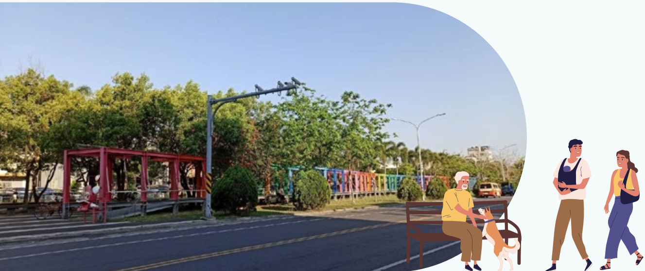
Coordinated with Sinying Art Park, the project created land for a park path and a combination park path and canal
