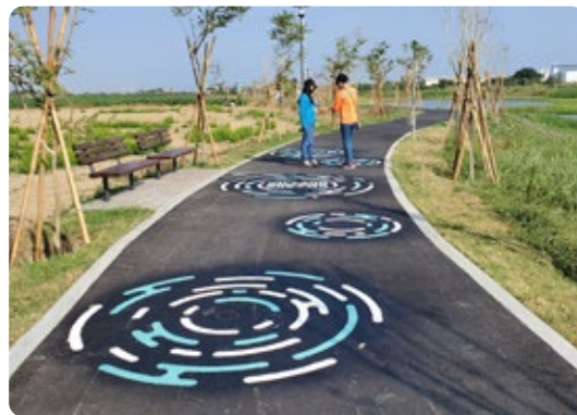
Results of Yuejin Harbor Park 18-3 and 18-5 waterfront path construction
