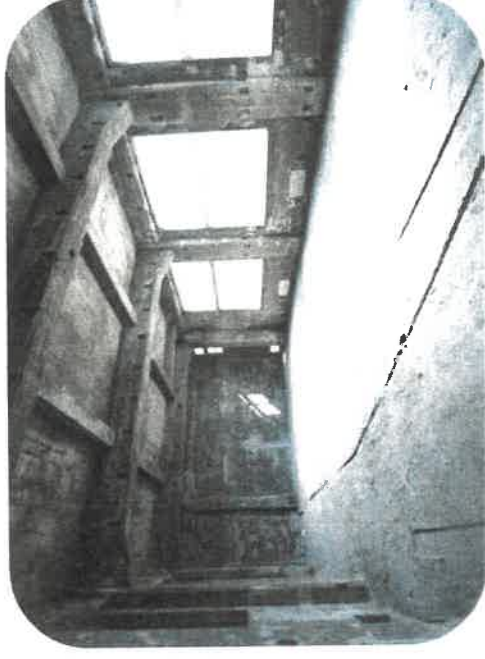
Second and third floor, unused during the "Manabikan" period
