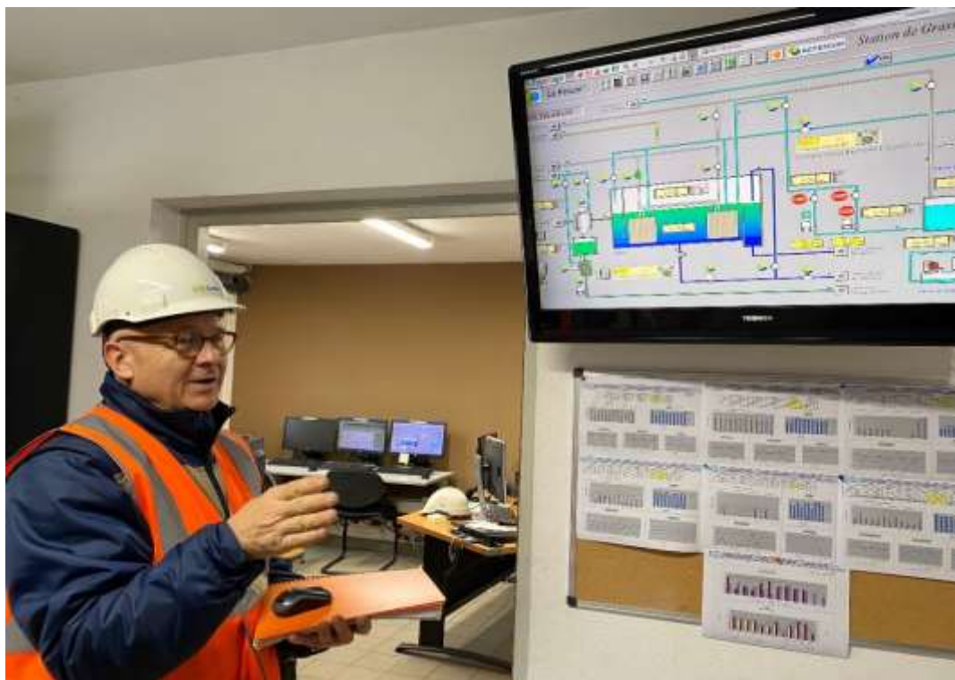
圖43 Grasse La Paoute MBR Plant 污水廠線上監控系統解說
