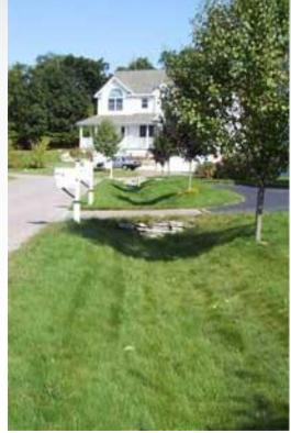
The bottom and sides of the swale must be vegetated. Surface ponding in a vegetated swale must not exceed 24 hours, however a longer time frame may be considered to match existing conditions hydrograph.
