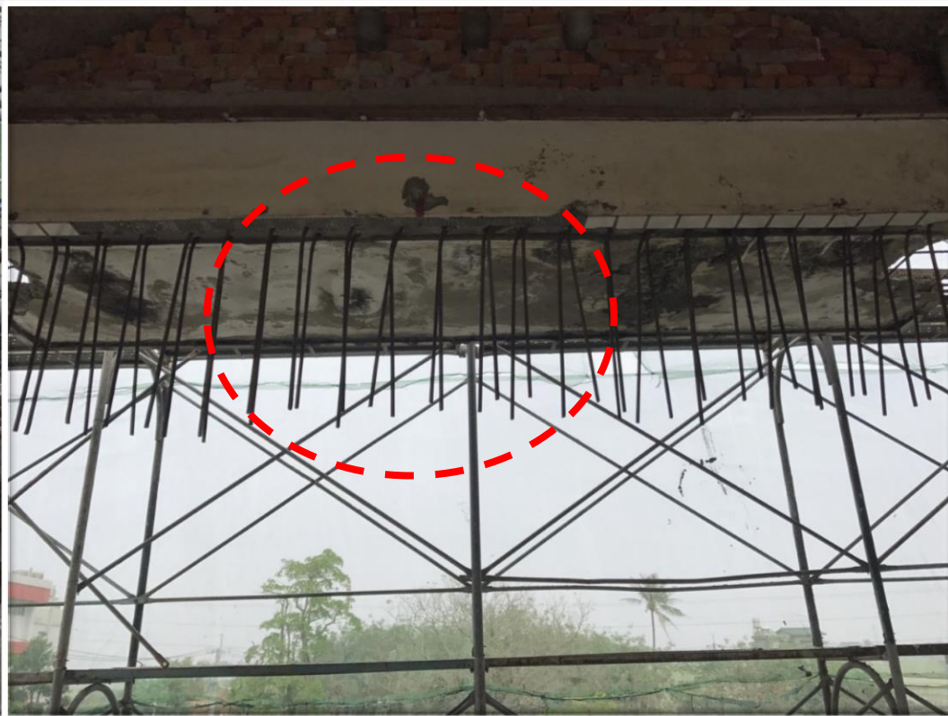
(C)二樓廁所(左棟及右棟)樑下剪力牆植筋後鋼筋超過1:6之斜度。【L】(5.02.99)
