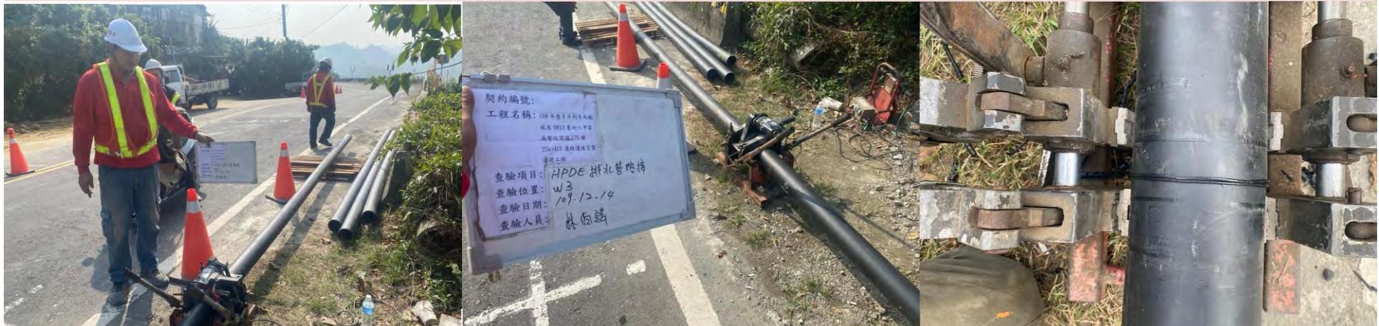
排水HDPE管採用熔接
